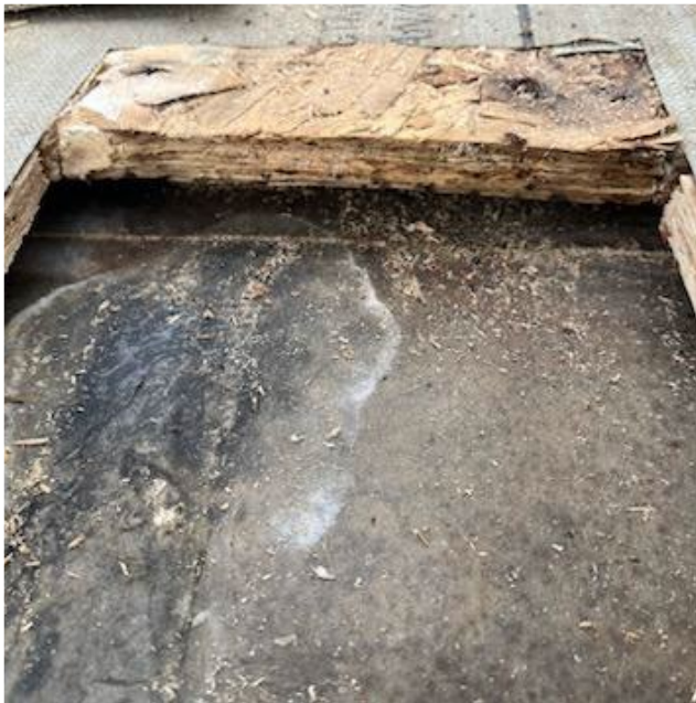
Roof Core pic #2
