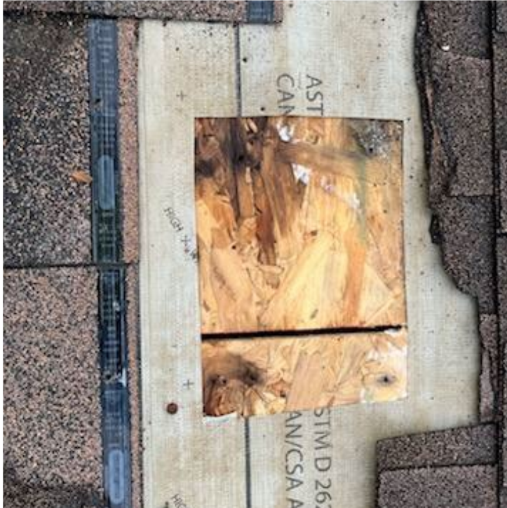
Roof Core pic #1
